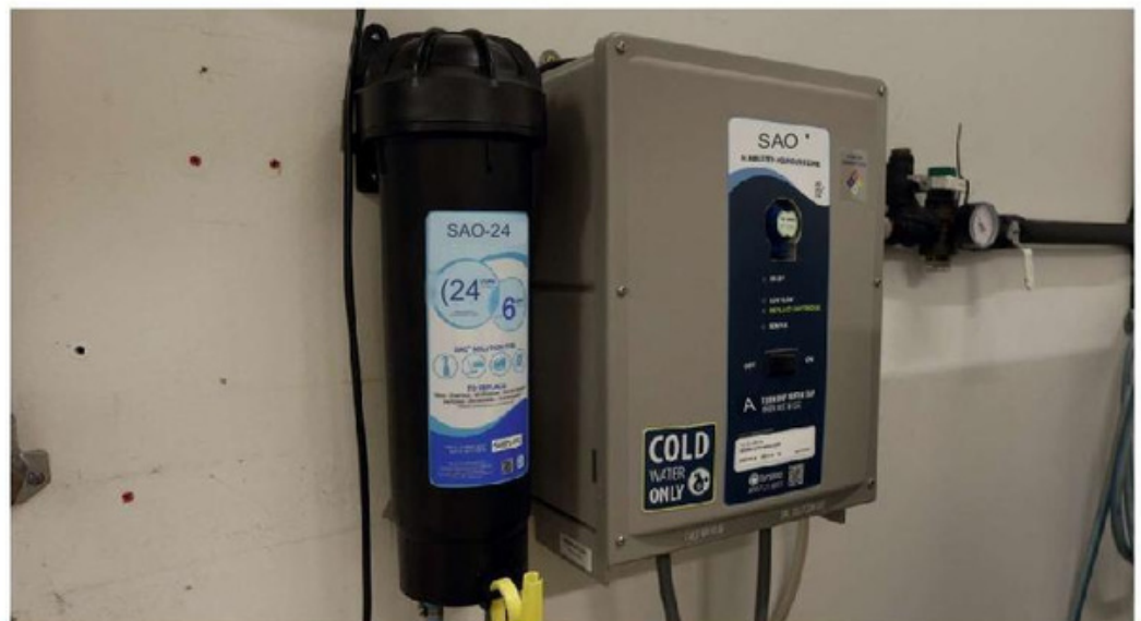
Tersano makes stabilized ozone water (SAO). This means that you can reduce the amount of chemistry.
