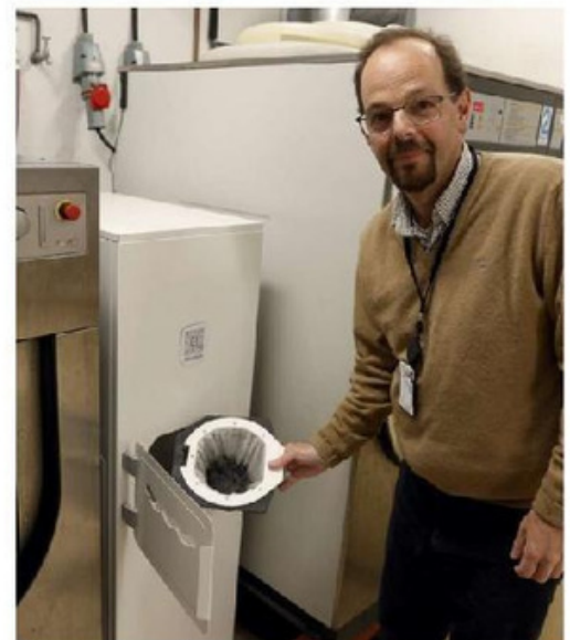
DSS has its own laundry for mops and cloths. Paulo Ruvina shows Mimbox, a solution that collects microplastics before the waste water goes down the drain.
